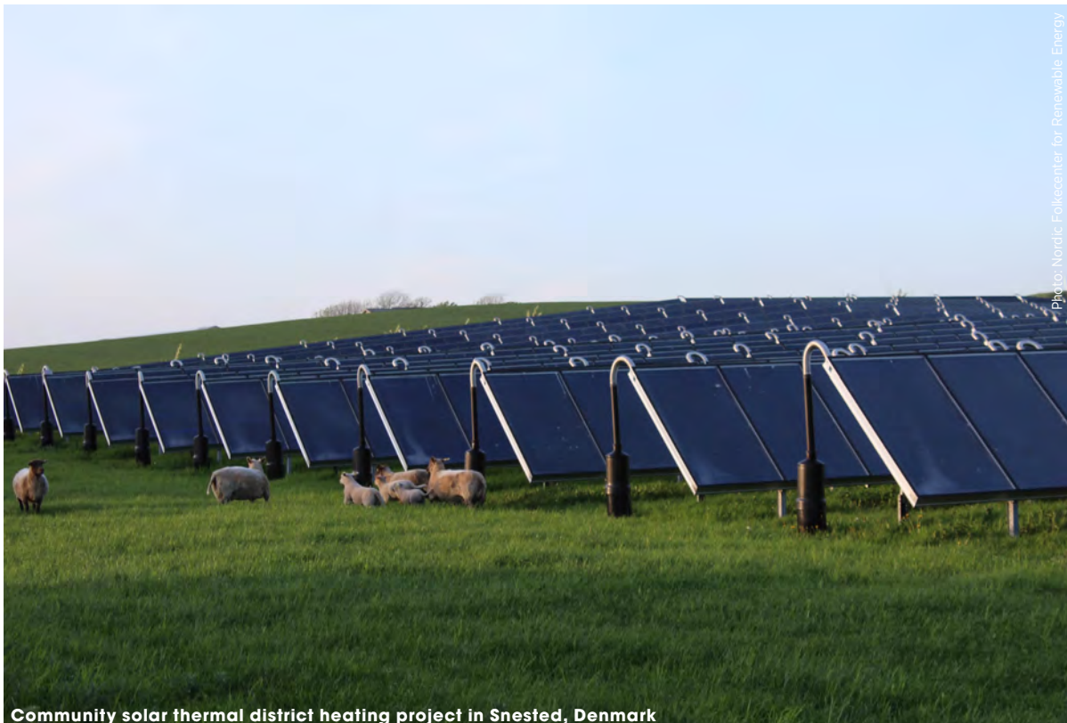
Community solar thermal district heating project in Sneksted, Denmark
