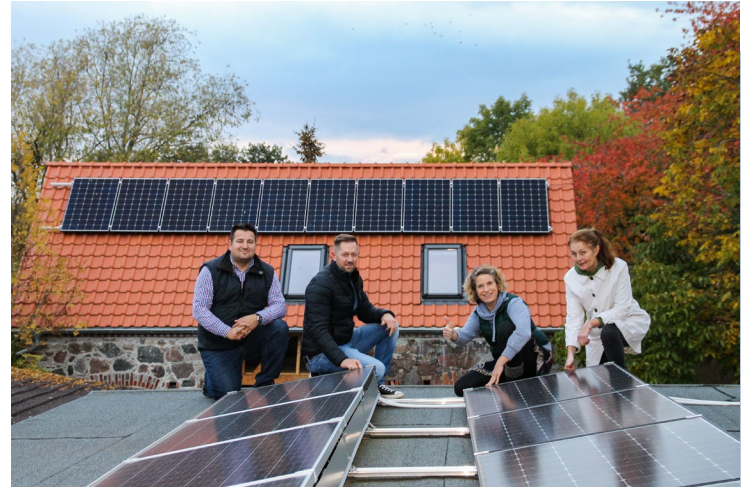
↪ First power plant for the kindergarden
