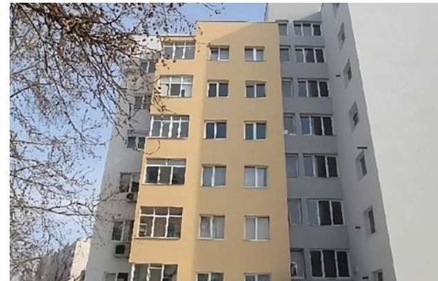
Building after renovation ©Asenovgrad Municipality
